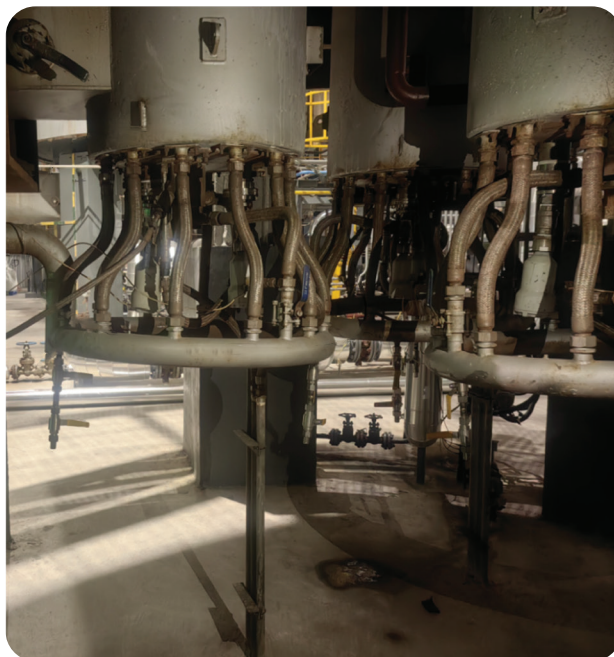
Figure: Vertical ring inlet system of benzene hydro heating furnace gas
